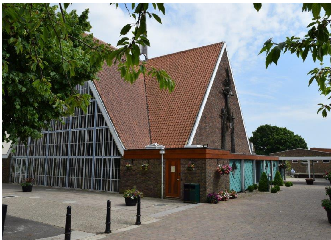
A locally Listed Building - The Chapel, University of Chichester, Bishop Otter Campus
